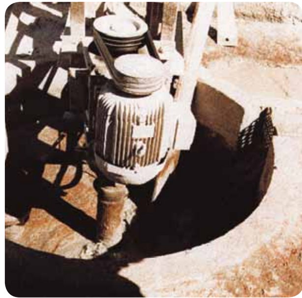
Photo 56. Waste pumping pit for final disposal
