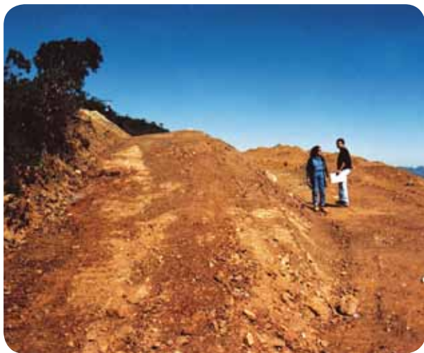
Photo 84. F2 after resloping for installation of a rainwater drainage system, followed by revegetation
