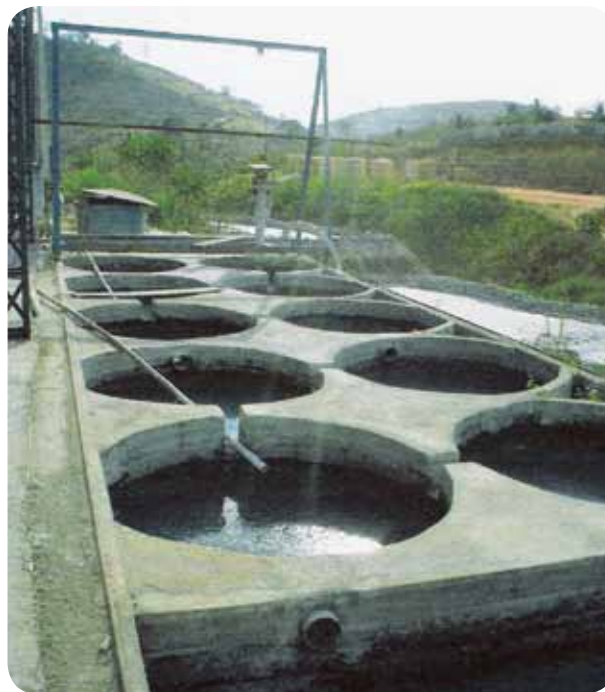
Photo 58. Effluent treatment system for waste from polishing processes. Source: Prezotti (2005)
