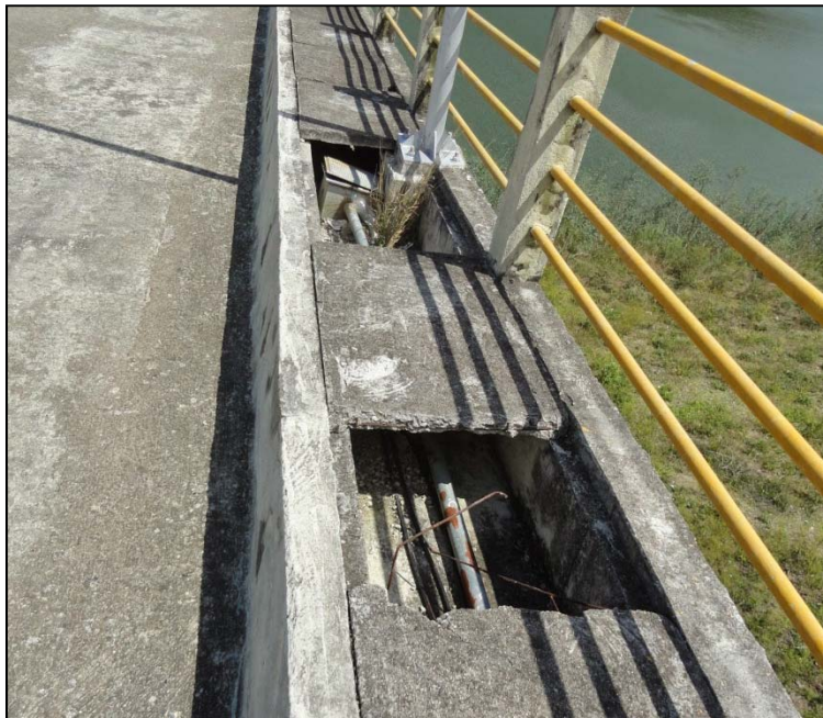
Figure 7: Minor maintenance issues such as cracking concrete at Jucazinho Dam may increase the need for costly electrical system repair or other major maintenance later.
